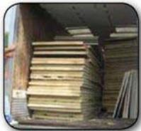
*Insulation board removed from a roof tear-off is stored in a trailer provided by Nationwide Foam and transported to a recycling center. (Photos courtesy of the EPDM Roofing Association.)*
